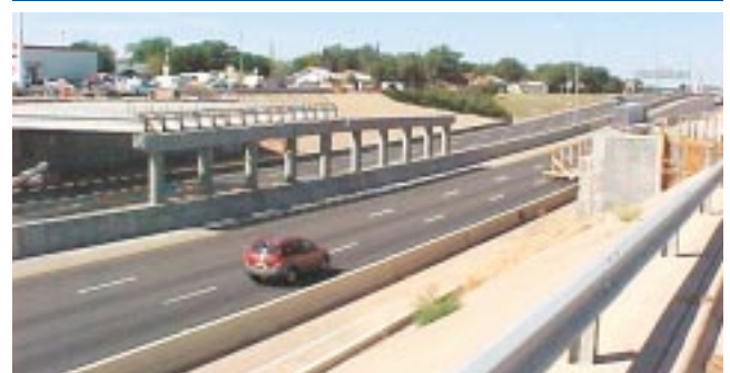
Bridge over I-40 – Amarillo, Texas
